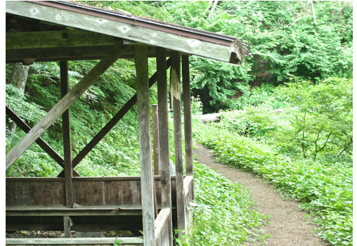
T11 / Teahouse shelter
